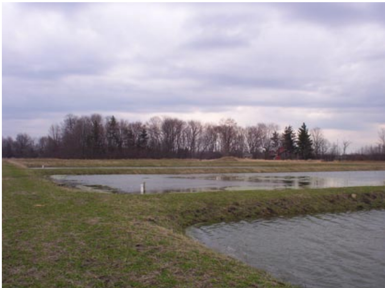
Figure 2. A photograph from the north bank of the wetland cells facing southeast. The protruding piping in each cell is connected to control boxes that will be used to maintain equal water levels in each wetland. This summer will mark the first growing and sampling season of the study.
