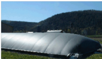
Figure 2b. A covered plug-flow digester, to help maintain temperature and protect from the environment (Kryzanowski).
