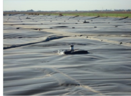
Figure 4. A covered lagoon at Oklahoma State University's Swine Research and Education Center
