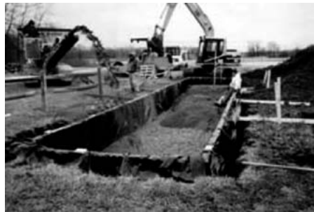
Figure 12a. A bioreactor built on-site.
